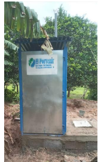
Sanitation facilities in San Antonio Camoapa
